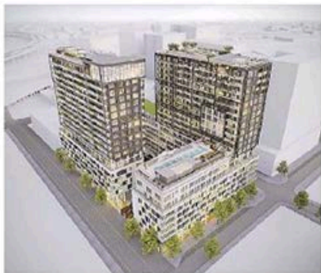
An aerial view of Lowney sur Ville, in Griffintown.
